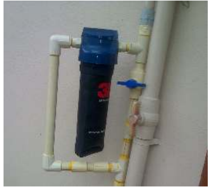
IAS141T installed at point of entry of flat
