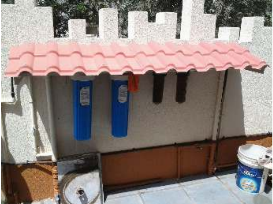
2 units IAS141T with a sediment pre filter and carbon pre filter for an independent house
