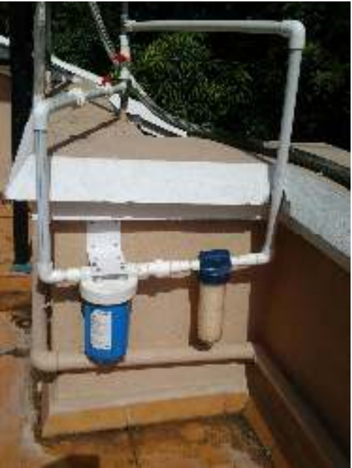
IAS141T with a pre filter AP801C for an independent house
