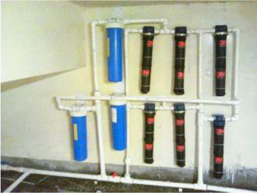
Centralized installation for 50 flats
