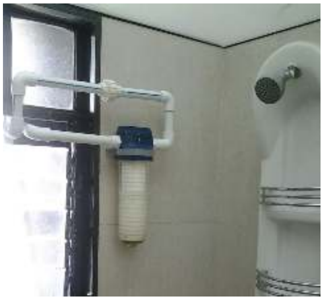
IAS141T installed in washroom
