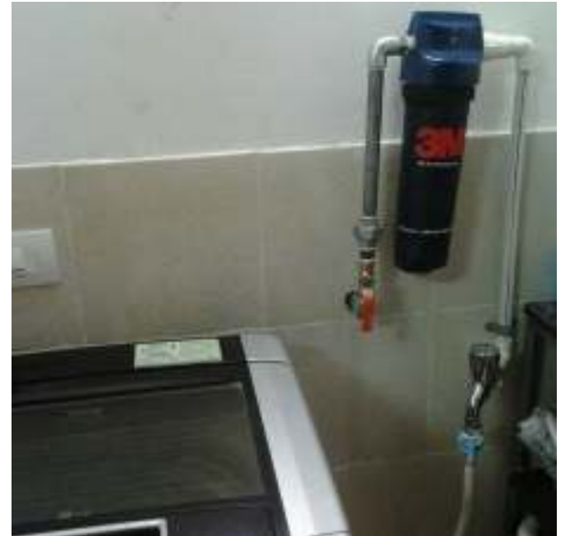
IAS141T installed in utility area
